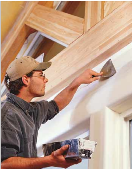
NO-COAT L Trim Install
